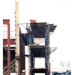
The ends of this scaffold are not properly guarded
