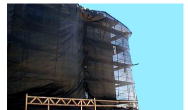
A covered scaffold has special wind load considerations
