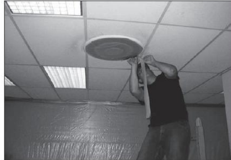
Sealing the ventilation system
