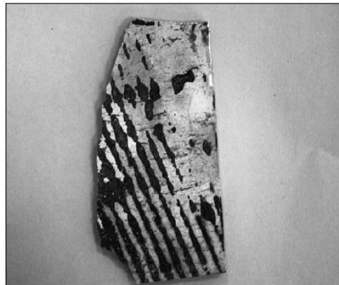
Vinyl asbestos flooring
